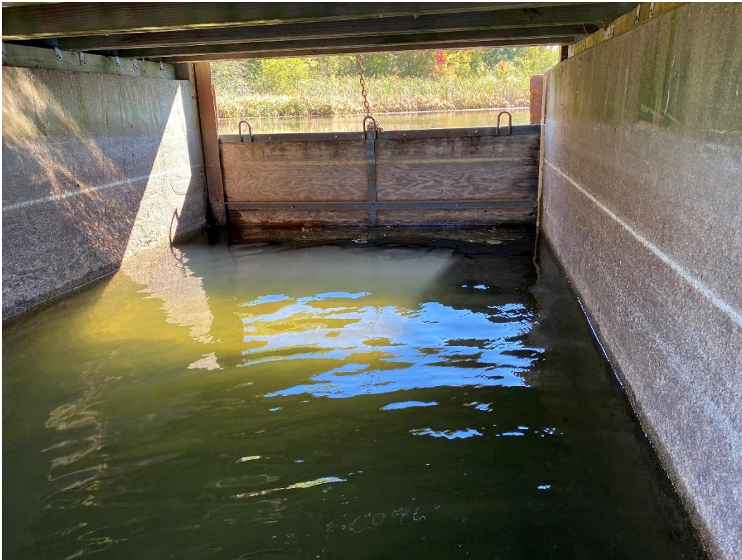
Far Right Spillway Bay
