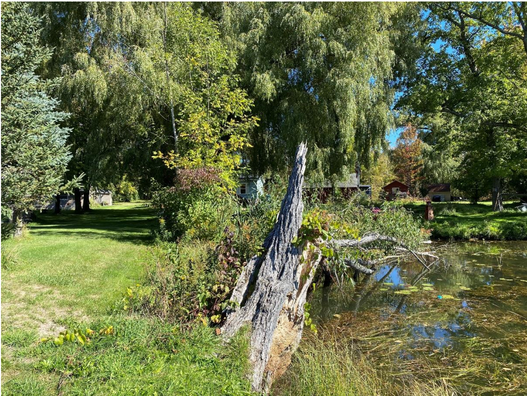
Dead/Down Tree on Right Embankment
