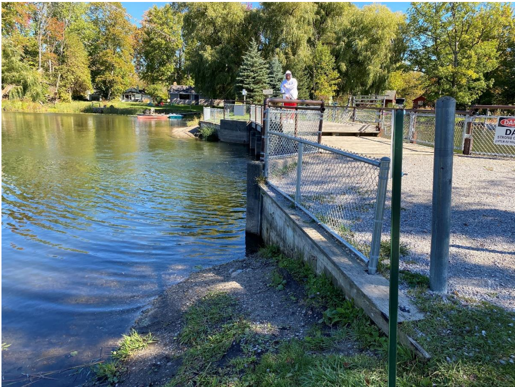
Downstream Side of Dam, From Left
