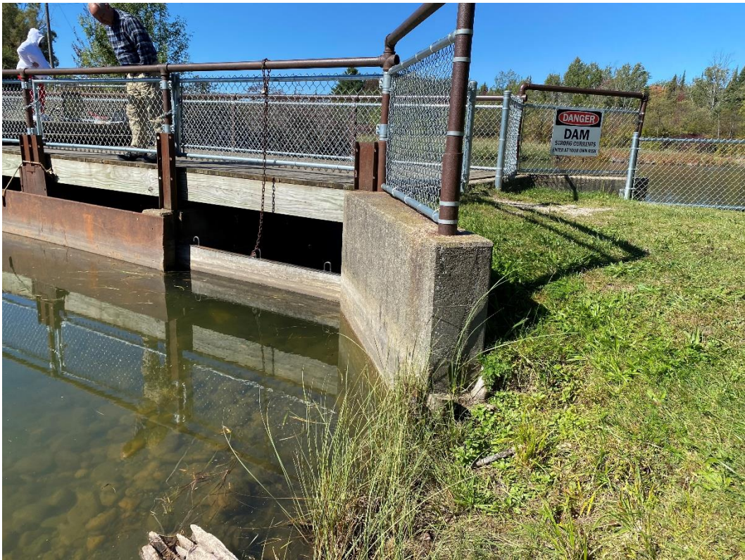
Upstream Right Wingwall
