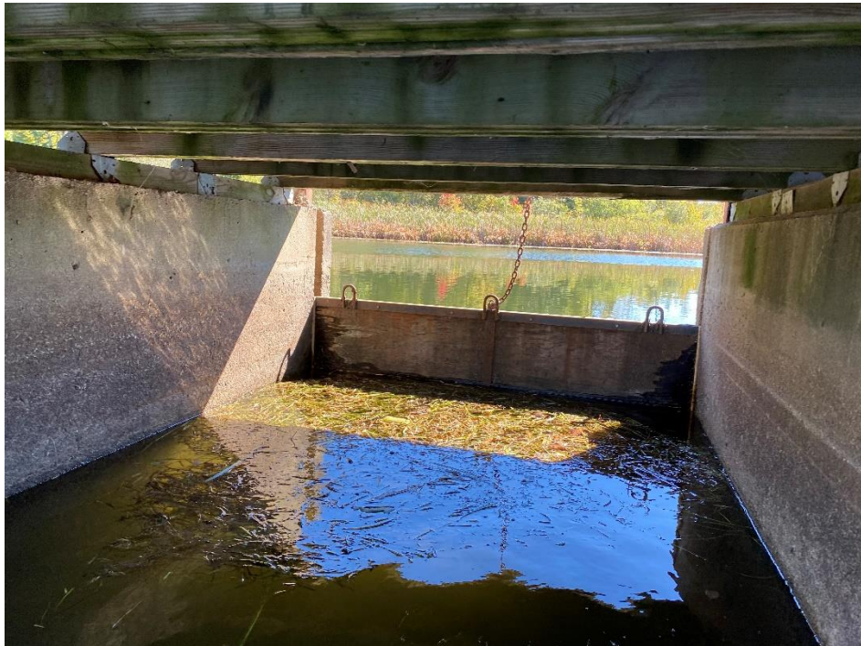
Spillway Bay, 2 nd From Left
