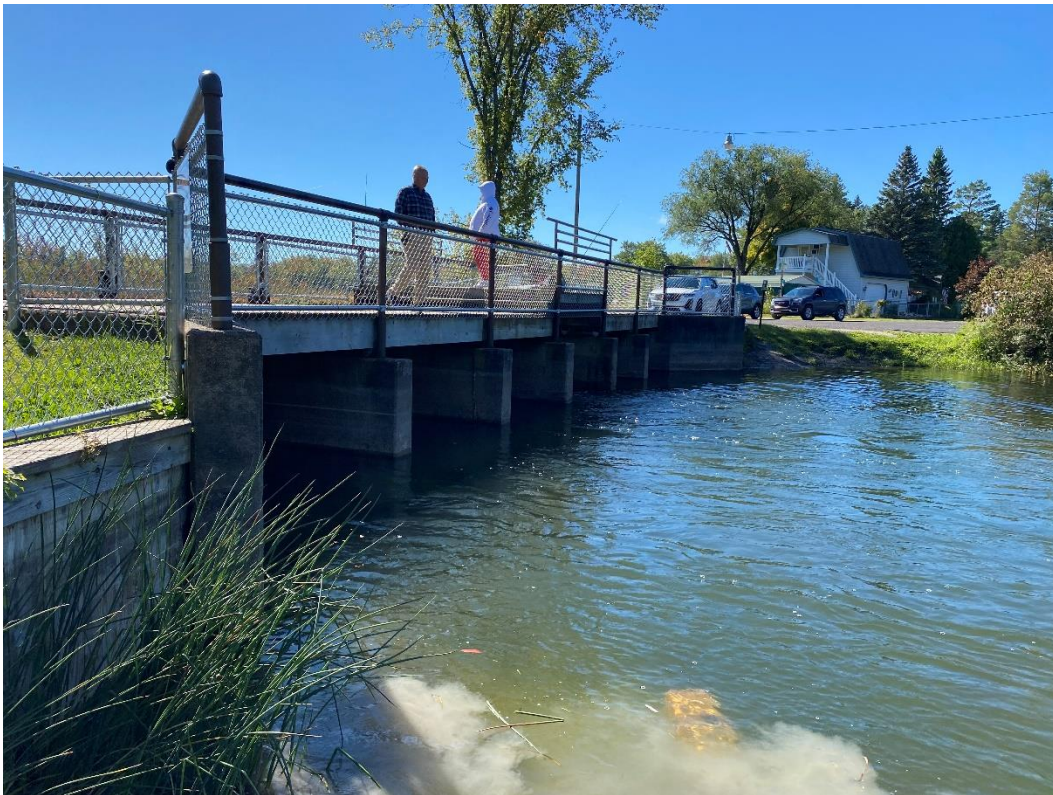
Downstream Side of Dam, From Right
