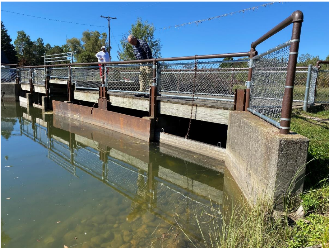
Upstream Side of Dam, From Right
