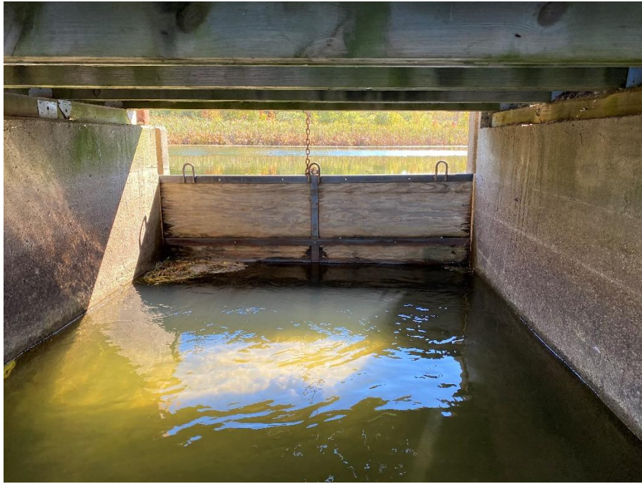
Far Left Spillway Bay
