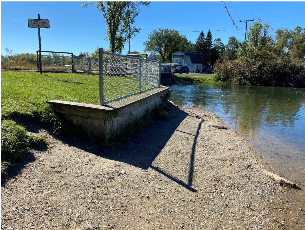
Downstream Right Wingwall
